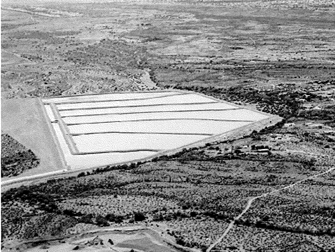
Figure 1: Recharge operations at a constructed facility in Arizona.
